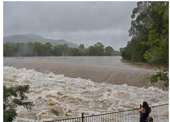
Black School Weir
